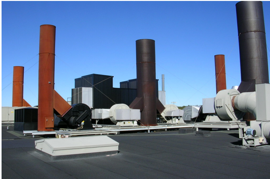
Figure 2 Typical environment on roofs of industries
