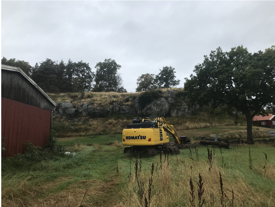
Figure 3.4: surrounding of the excavator
