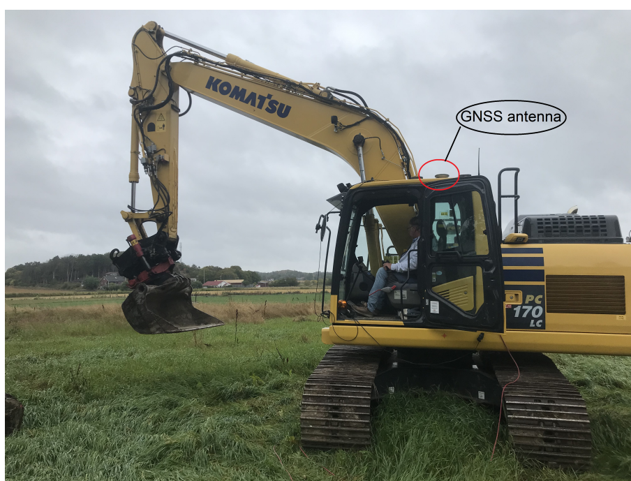
Figure 3.1: Placement of the GNSS antenna on the Excavator
