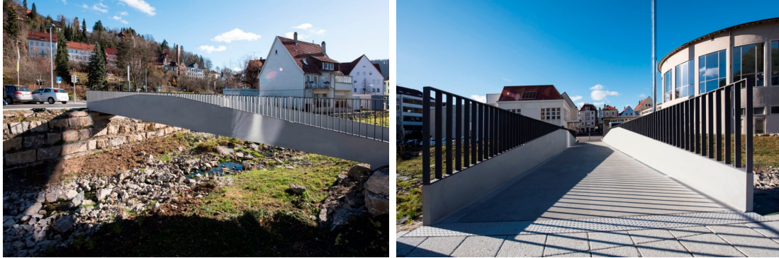
Figure 2.10: Photographs of the Albstadt-Ebingen bridge © solidian GmbH (Solidian-Kelteks, n.d.-a)
