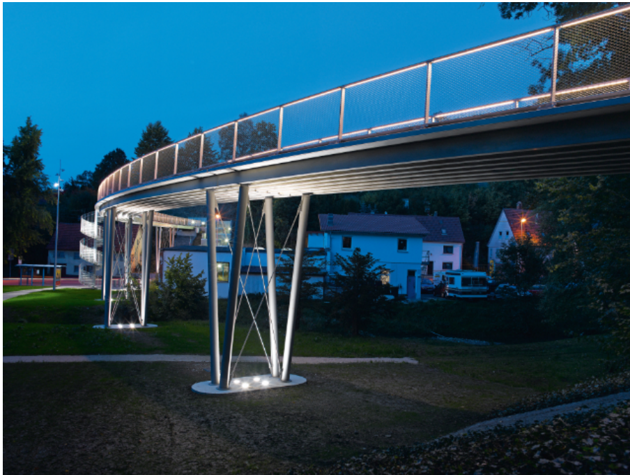
Figure 2.9: Photograph of the Albstadt-Lautlingen bridge © solidian GmbH (Solidian-Kelteks, n.d.-a)
