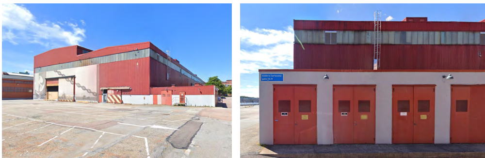
Fig 10& 11 A large warehouse (parking lots nowadays)
