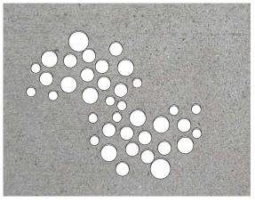
The circular and elliptic holes arranged in an irregular pattern contrast to the existing openings in the tower that are very orthogonal and function driven.
