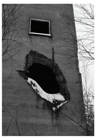
There are two different kinds of openings in the existing facade, the rectangular openings that used to contain windows and the organic holes caused by the passage of time and wear of the concrete. The chosen solution can be used for both types.
