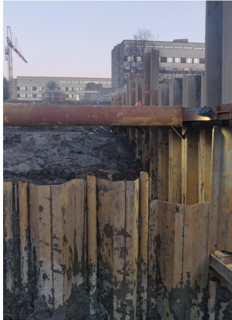
Figure 2.1: Sheet pile structure with associated stabilizing member.
