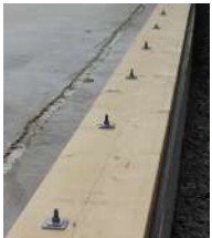
Sill fixed in base with sill nail.
