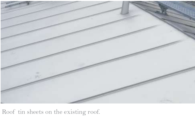
Roof tin sheets on the existing roof.
