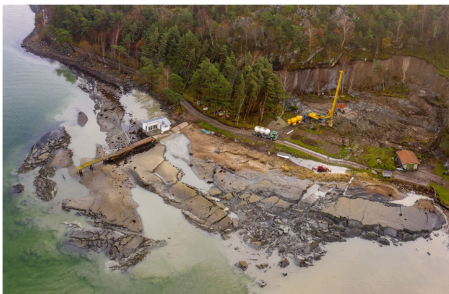
Figure 2.4: Photograph over the area of the landslide [12].
