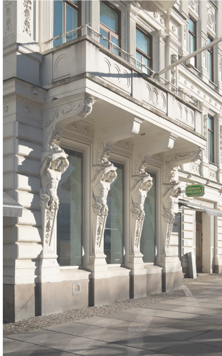
Sculptural facade of varying depth, articulated entablature, vertical wooden windows between rhythms of pilasters.
