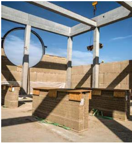
Image 17. The Ricola warehouse, Construction (© Markus Bühler)
