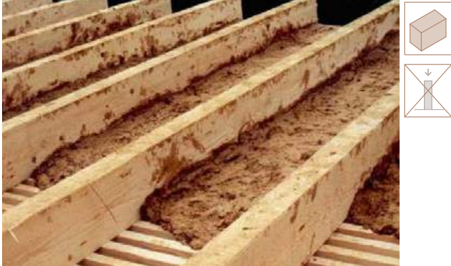
Image 33. Loam deck infill (Photo : Walter Unterrainer)
