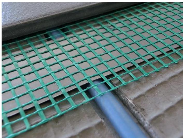
Figure 6.1 Placement of graphite grid in floor heating system
