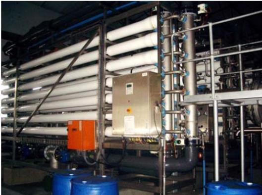
Figure 6 A membrane rack with membrane modules. Photo: Helen Ander.
