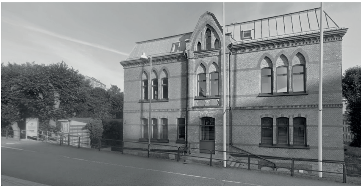
9. Facade from Chalmers tram stop
