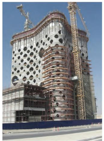
Fig. 24, "O-14", office tower in Dubai, external reinforced concrete structure, construction, Reiser & Umemoto
