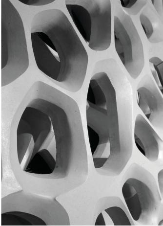
Fig. 25, "Cocoon Club", panellised concrete wall, design by 3deluxe, development of concrete elements by Villa Rocca
