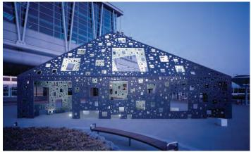
Fig. 29, "Shin Yatsushiro Monument", pre-cast walls and cast in place roof, 7cm thick glass fibre-reinforced concrete, Kumiko Inui
