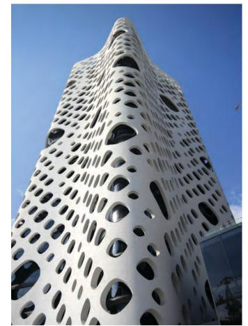
Fig. 23, "O-14", office tower in Dubai, external reinforced concrete structure, Reiser & Umemoto
