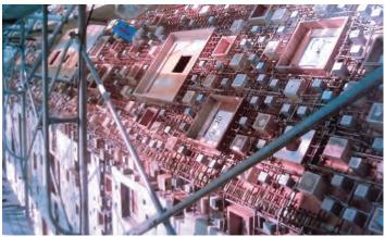
Fig. 30, "Shin Yatsushiro Monument", pre-cast walls and cast in place roof, 7cm thick glass fibre-reinforced concrete, roof casting process, Kumiko Inui
