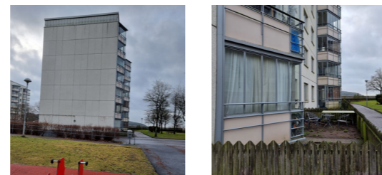
Fig. 58. Windowless façade and closed blinds.
