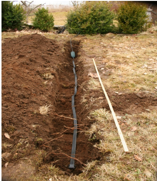
Figure 17. 3 meters cable, Aquaflex humidity sensor.
