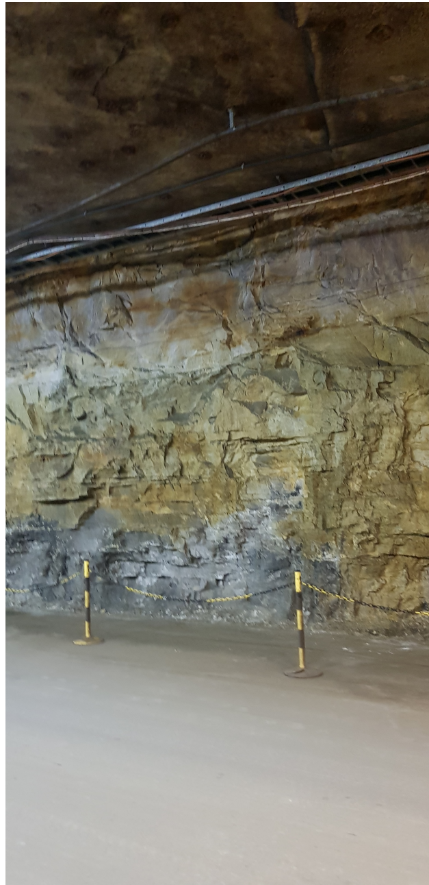
Figure C.1: Inside one of the main corridors in the Kvarntorp mine. Sandstones layers SL4 and SL5 are visible
