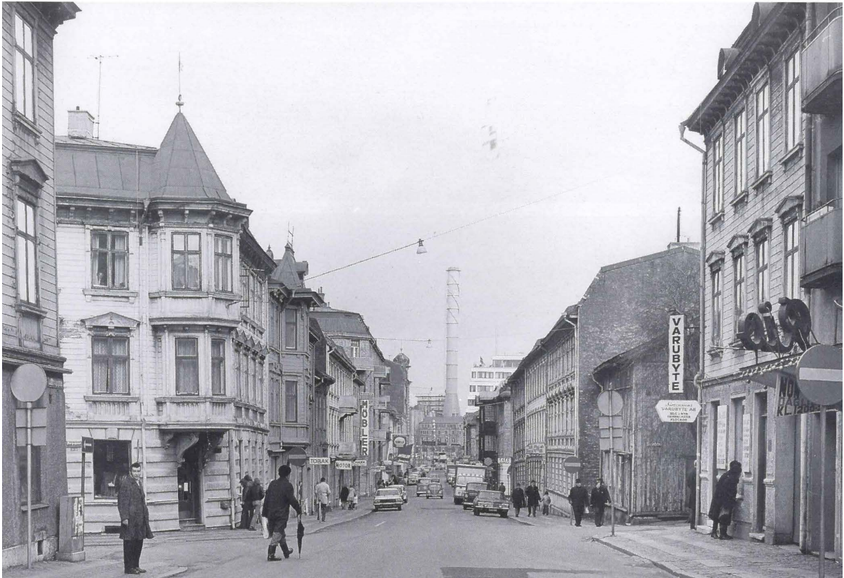
Figure 4: view from Landsvägsgatan towards north and Rosenlundsverket, 1973.
