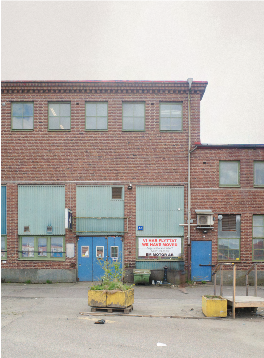
Part of current northern facade
