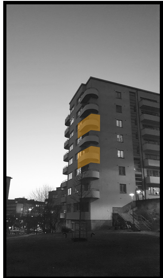
Spaldingsgatan 15A, Gothenburg: Projecting balcony over a corner was popular in the 30s. Mainly for the appearance but also generates a wider field of view and can create a stronger interior connection through sight.
