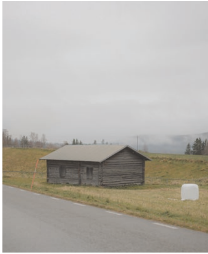
Original log timber structure
