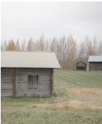
Original log timber structure
