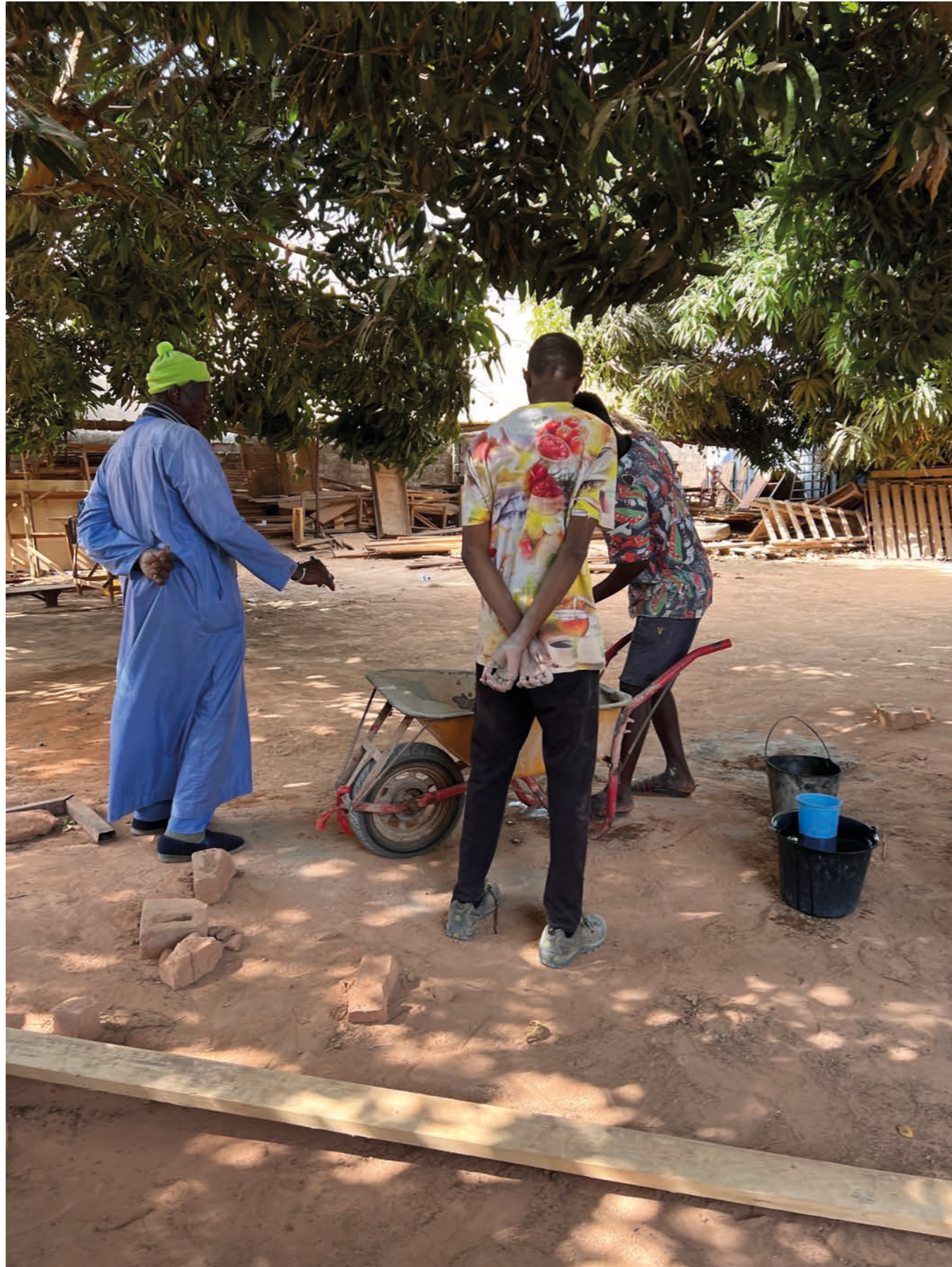
Mixing the mortar
