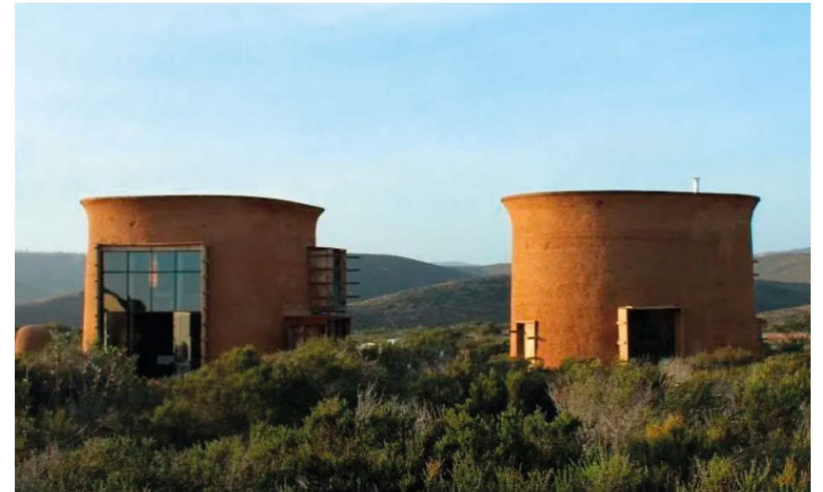
Galeria 2 Hijas in California, built out of cob in 2021 by Cla Clá (n.d.)
