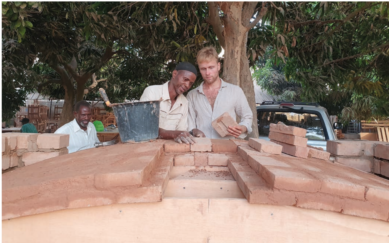
Fitting the final piece: the key stone.
