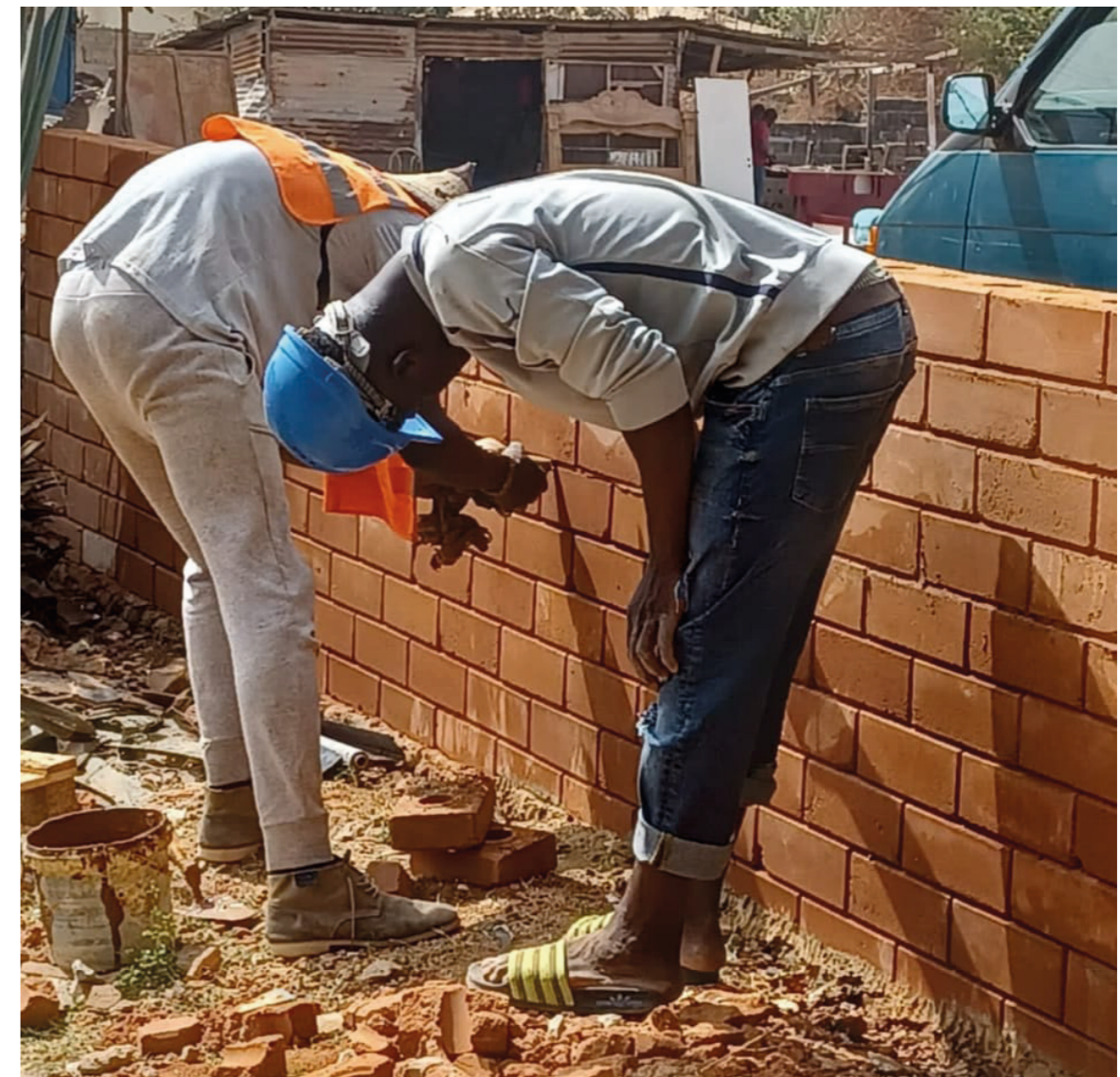
Plastering the brick joints of a compressed earth blocks wall in Kanuma, The Gambia.
