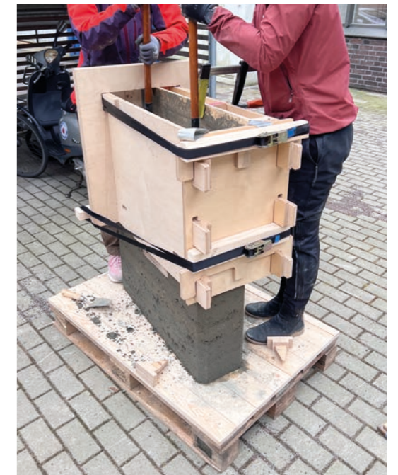
Shifting the formwork upward
