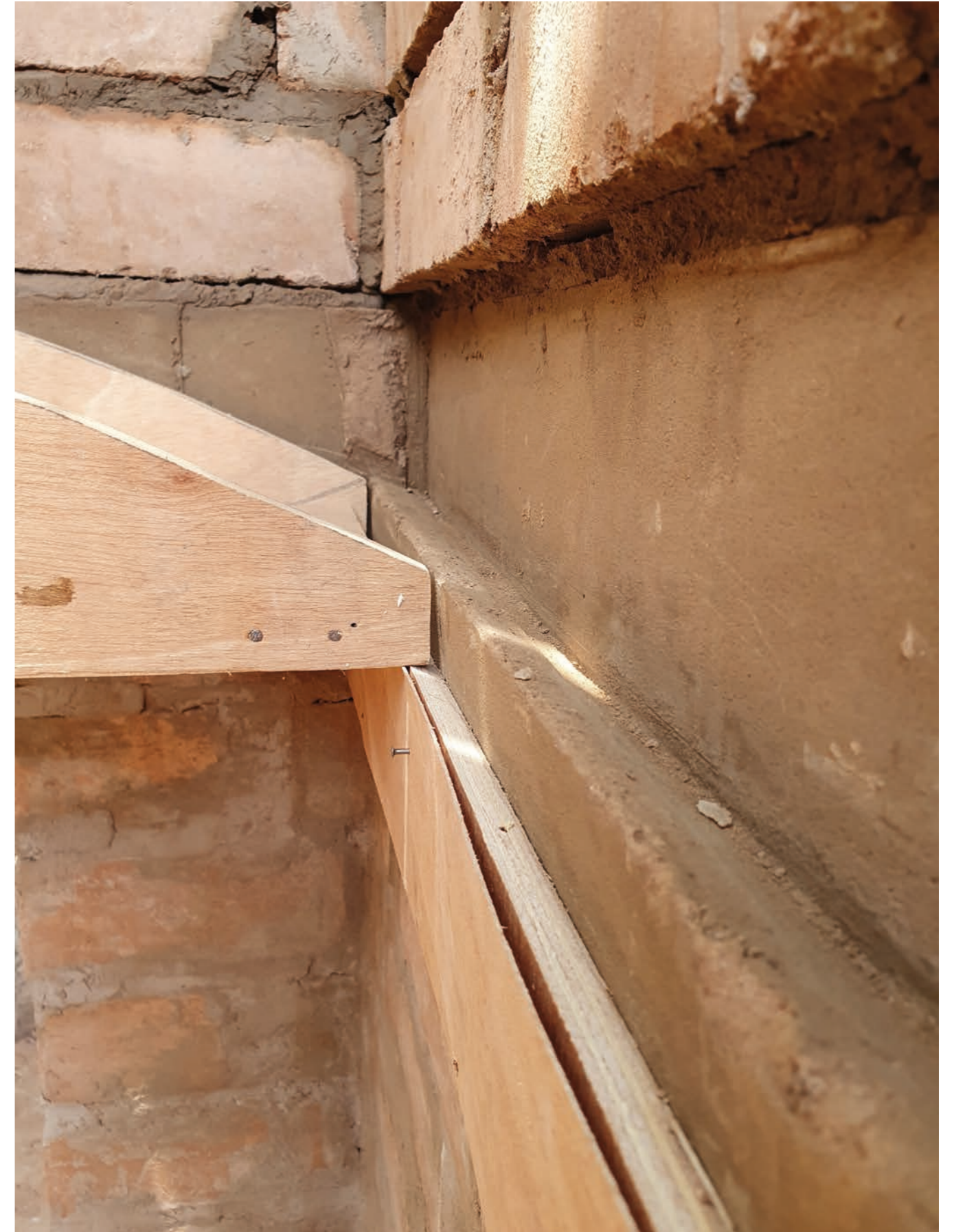
Aligning the formwork for the vault.
