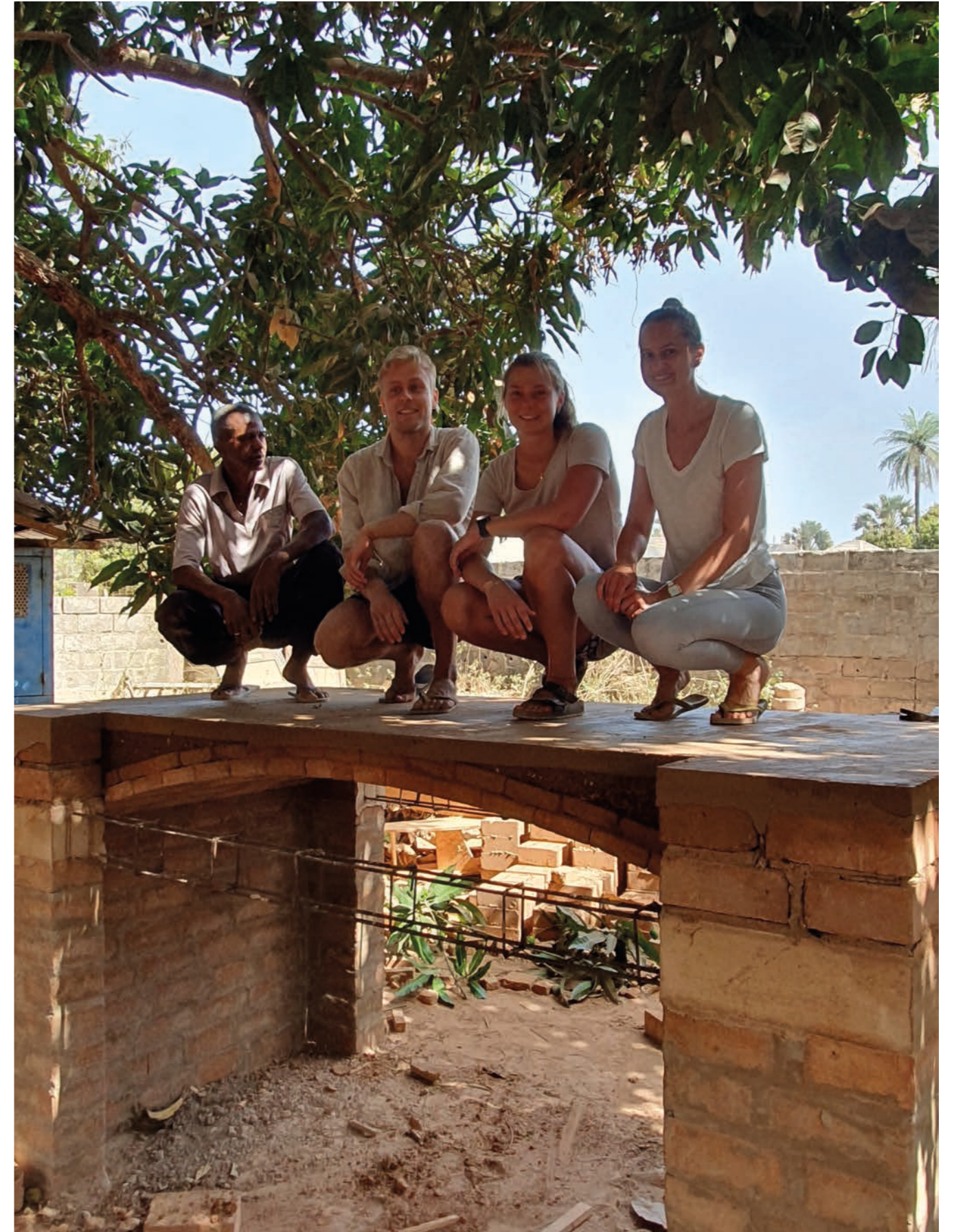
Finished floor slab – it held!
