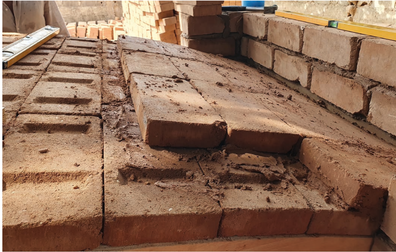
Progression of the vault
