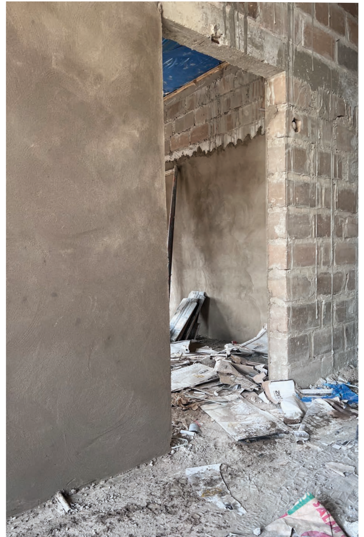
The rough concrete blocks surface is plastered for a fine finish
