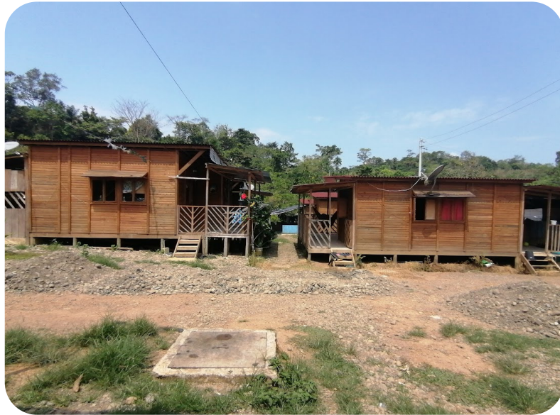
Self-built house expansion in Becuarandó
