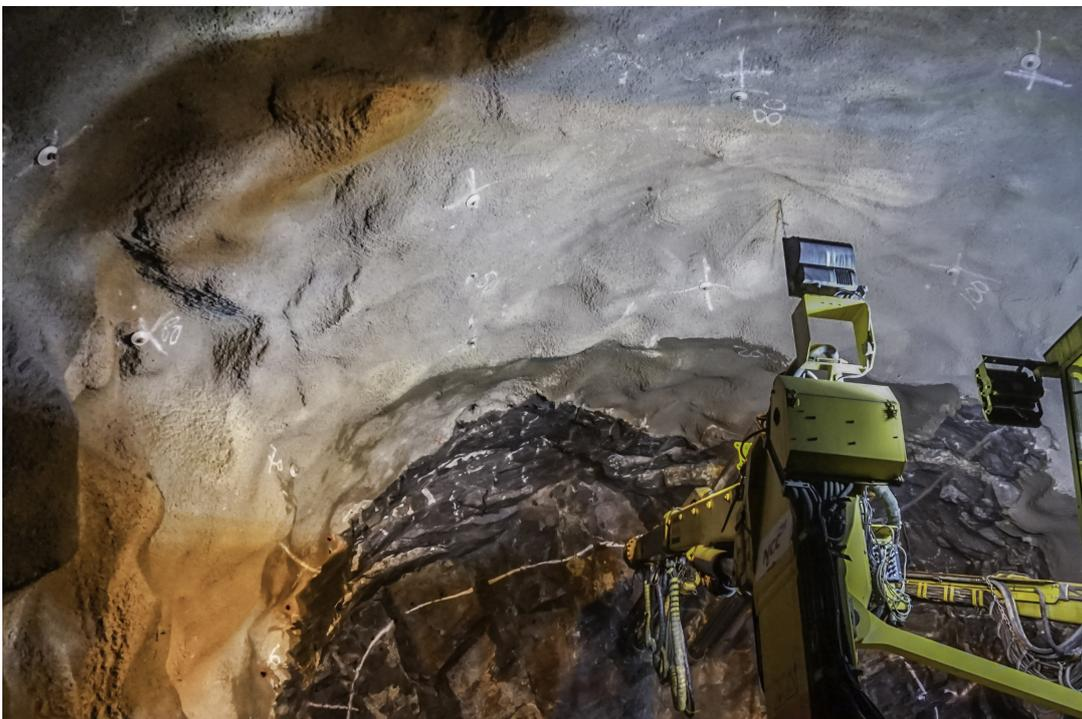
**Figure 5.12:** Closeup of the bolting and drilling machine in the Västlänken tunnel, station Korsvägen
