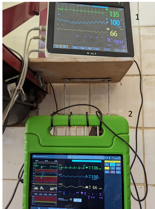
Figure 2.1: The main part of the Impala system. On top (1) is the bedside monitor displaying the vital signs with attached wires, and on the bottom (2) is the bedside tablet with the GOAL 3 app.
