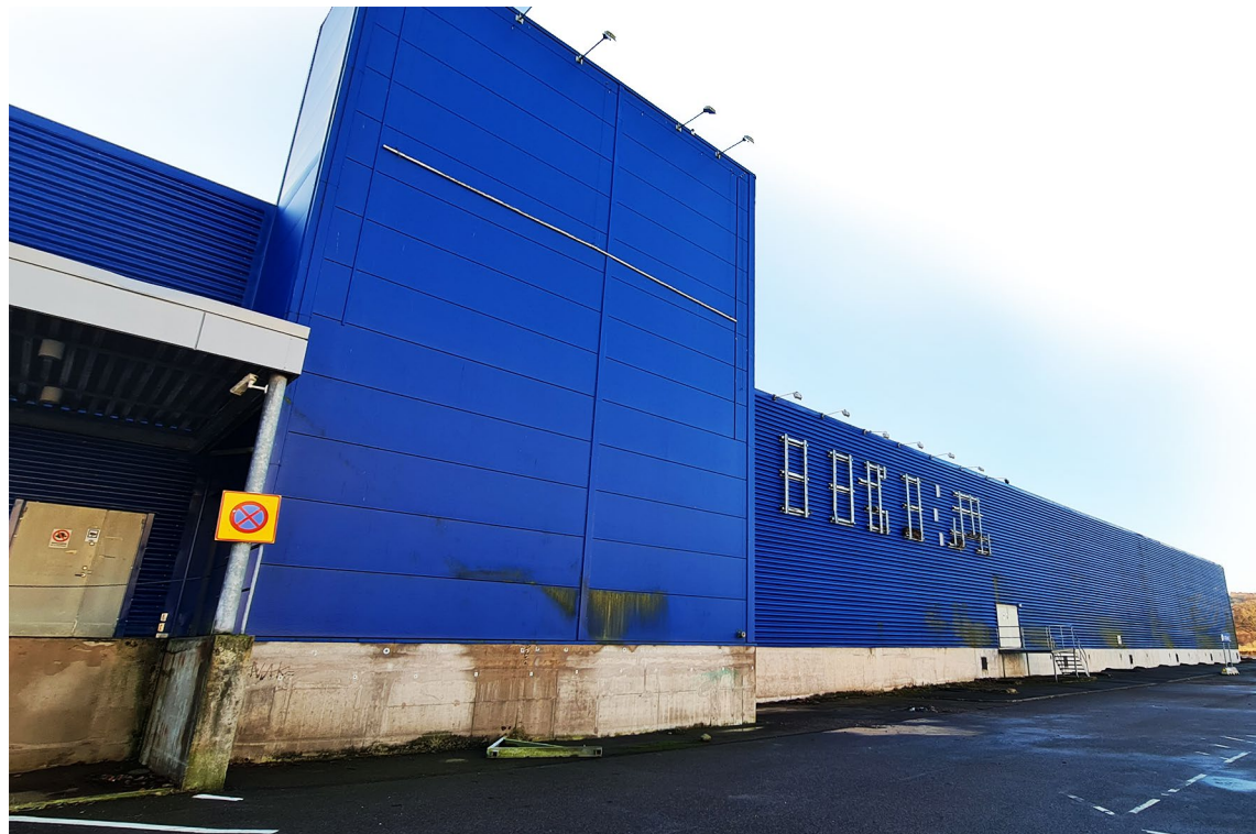
Figure 11. Current view of the north facade, 2023.
