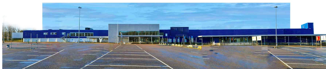
Figure 10. Current view of the east (entrance) facade, 2023.
