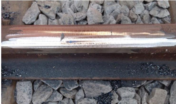
Figure 1.8 - Appearance of the repaired area after grinding [10]
