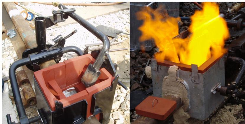
Figure 1.3 – HR process – mould preparation (left) and preheating phase (right) [2]
