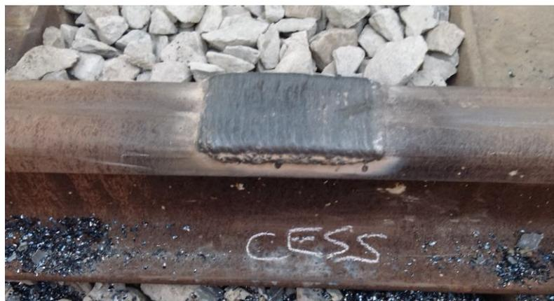
Figure 1.7 – Appearance of the repaired area after the third layer is laid [10]
