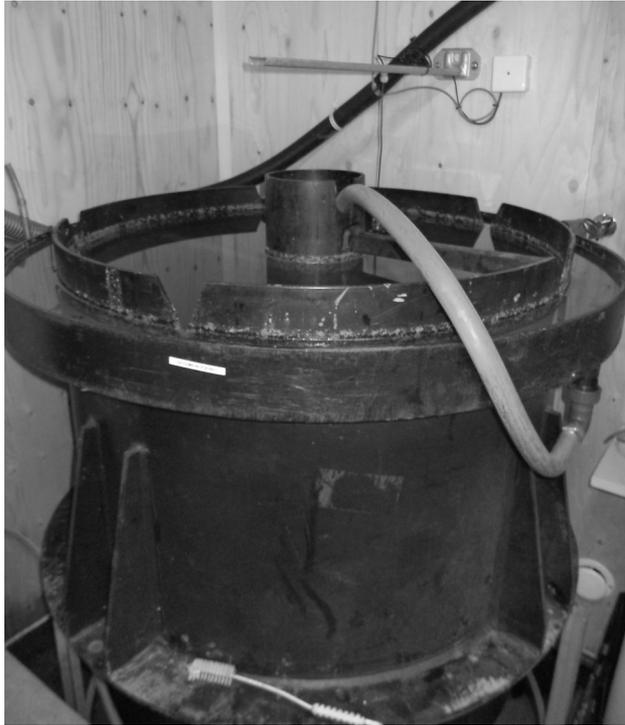
*Figure 6.9 The sedimentation tank at Brudaremassen pilot plant 2015*
