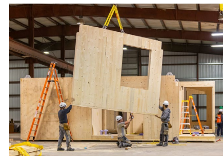
image 81. Bearing Walls construction
