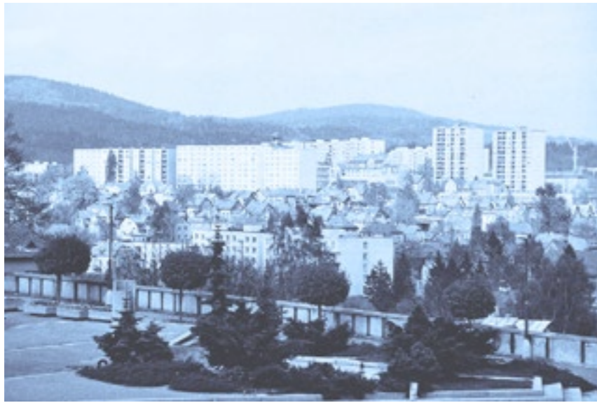
figure |12 View on the Šumava estate from the square
