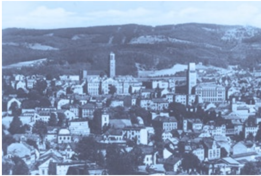
figure |13 View on the city centre, city of Jablonec
