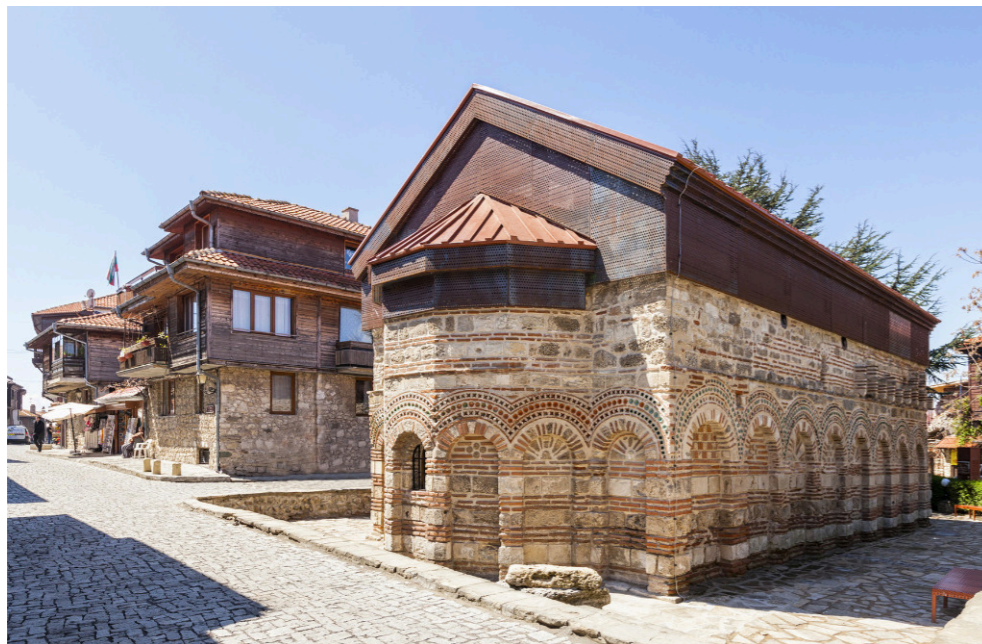
Source: https://www.archdaily.com/573012/conservation-restoration-and-adaptation-of-church-st-paraskeva-te-architects (access 17/10/2023)
