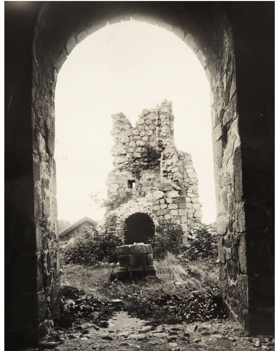
The ruin before the extensive restoration carried out in the 1890s. View from the central tower towards the nave and the west tower. The ruin is nestled in greenery and the central pillar appears to be leaning and missing several stones in the lower parcels. Unknown year. Source: Bjerking AB. (2020, June 23). St Per - restaurering. p.4.
