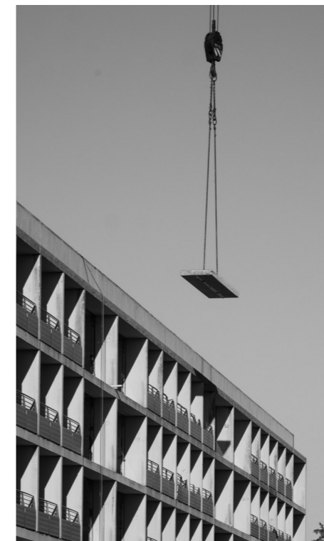
Fig. 5 Dismantling of HC element. Image source: GXN
