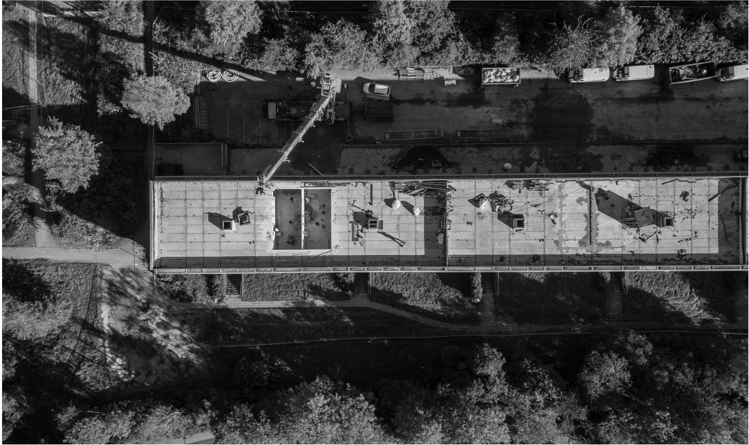
Fig. 10 Dismantling of HC elements in Gellerup. Image source: GXN
