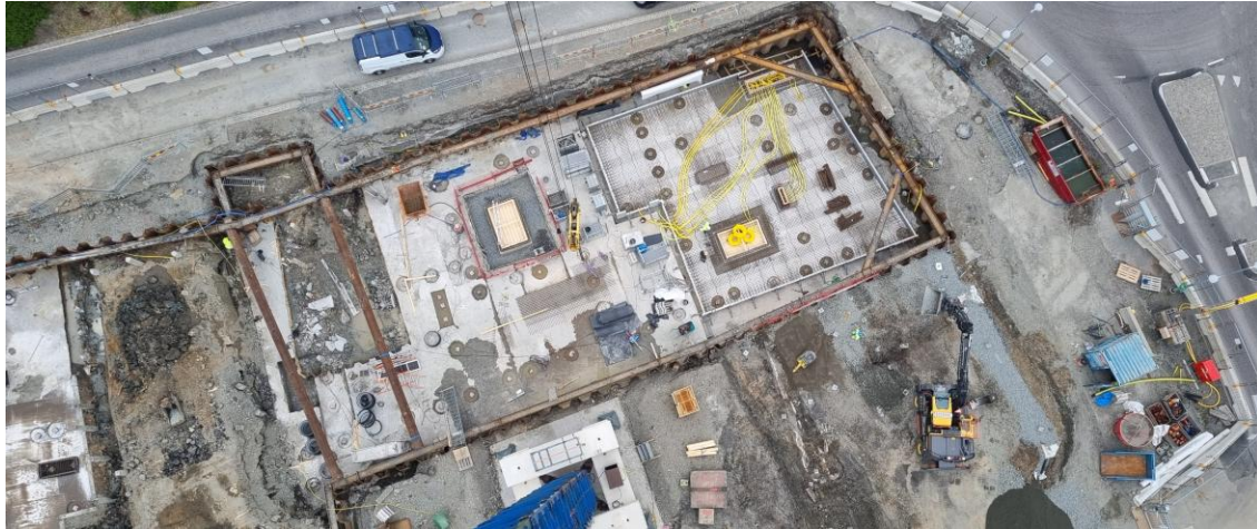
Figure 15: Earthworks phase at Solhöjden. (JM, 2025a).
