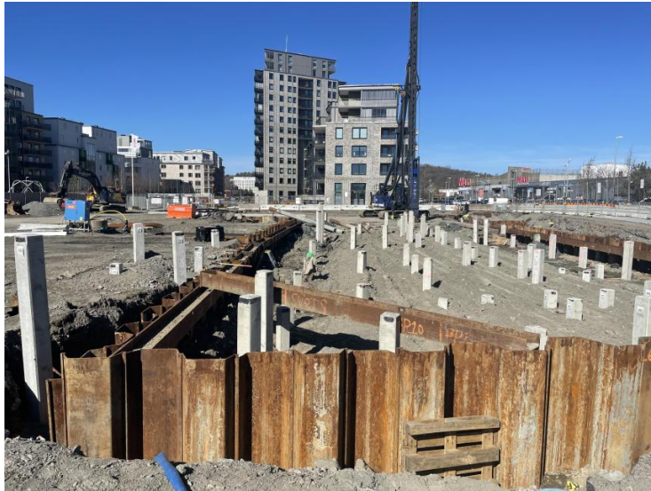
Figure 17: Foundation work, including concrete piles and steel sheet piling. (JM, 2025b).
