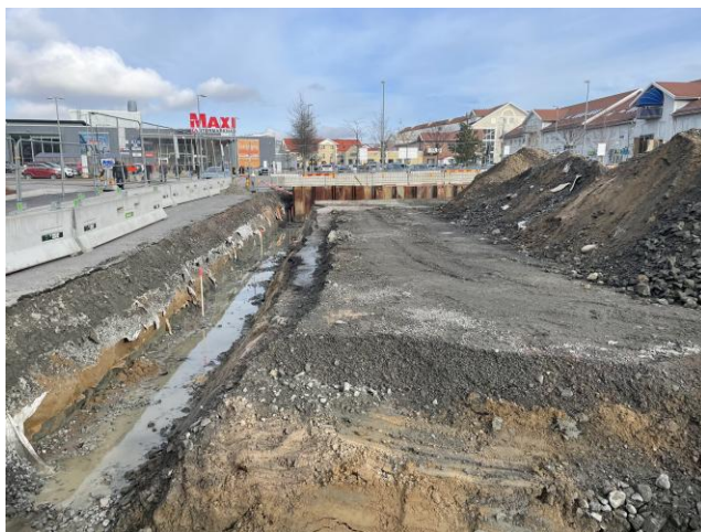
Figure 10: Solhøjden during the earthworks phase. (JM, 2025d).
