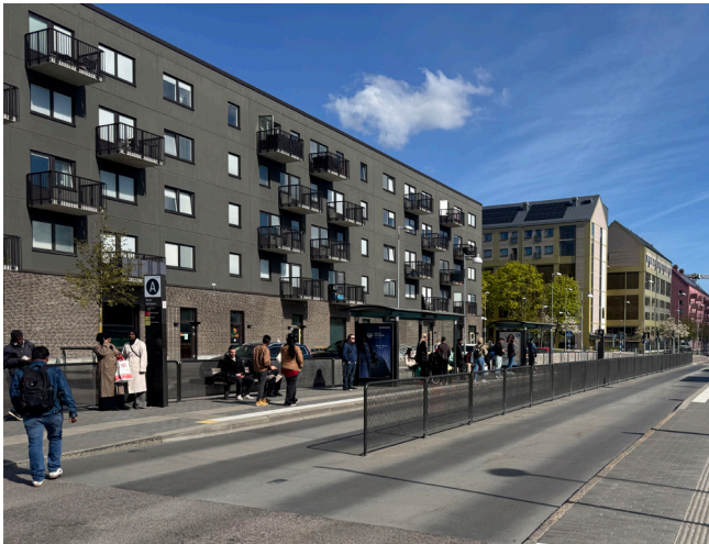
Fig. 30: View of Litteraturgatan.
