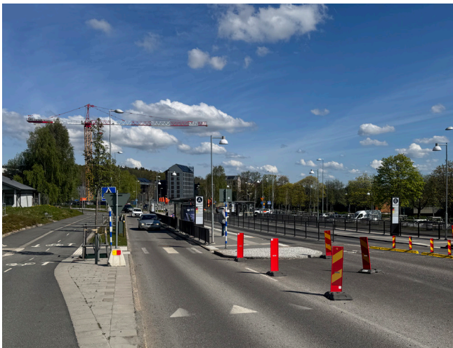
Fig. 31: View of Litteraturgatan.
