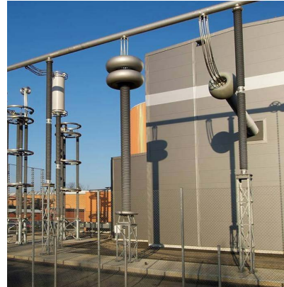
(b) Post insulators consisting of load bearing insulator tubes made of epoxy resin and fiber-glass and housing made of silicon rubber.
