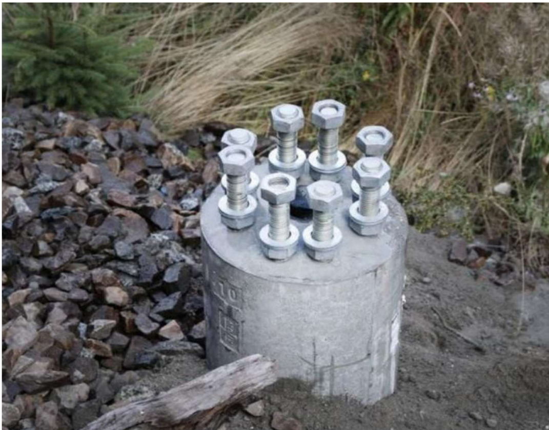
Figure 6: Mofix 1 foundation pillar installed example.
