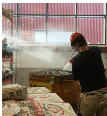
Adding about 60L water to the mix.
