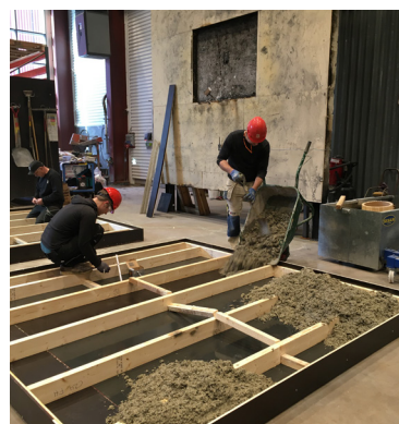
The mixture is poured in the framework.
