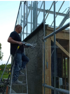
Image 27. Spraying the hempcrete
