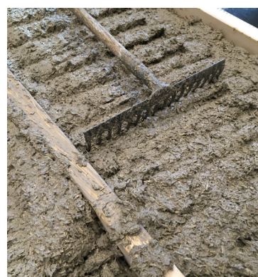
Zoom on spreading of hempcrete. A rack was used.
