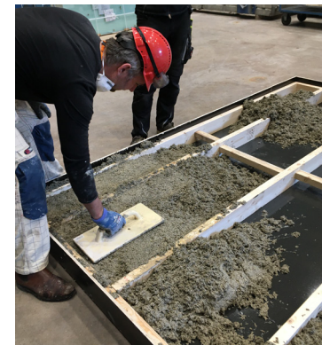
The hempcrete is tamped, important not to apply too much pressure.
