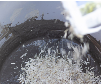
Adding the hemp shivs to the clay-slip.
