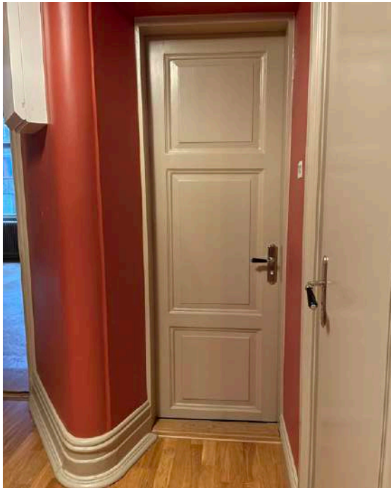
Image 49. The hall on the west side, a perspective outside the washing room with the repaired original doors.
