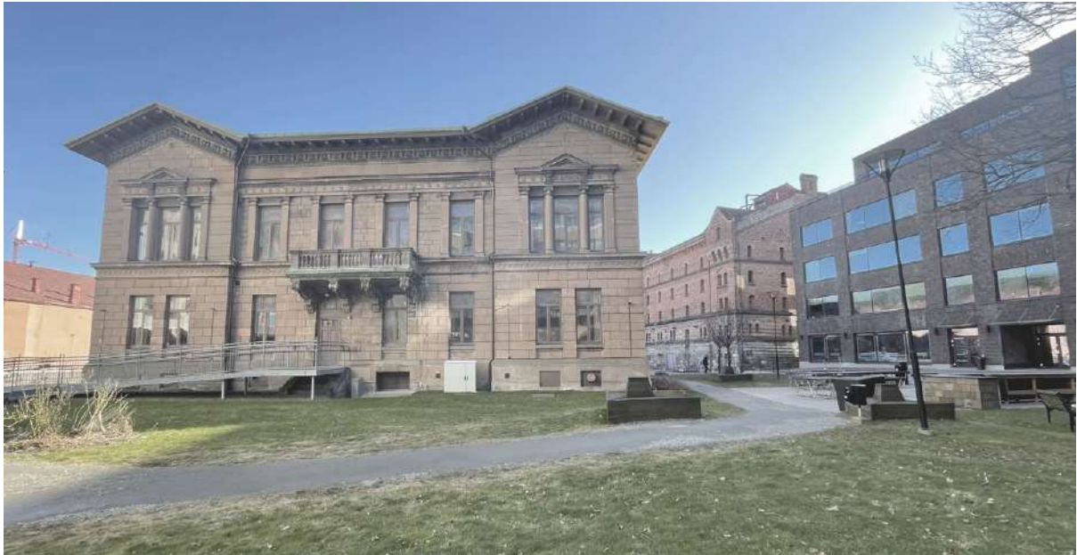
Image 23. North facade with the added ramp.
