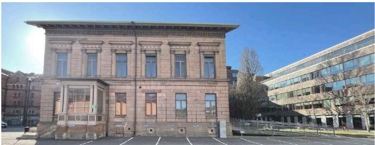
Image 24. East facade with the added ramp.
