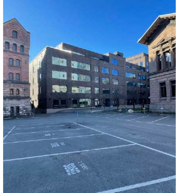
Image 14. (d) View from the parking on the south side.
