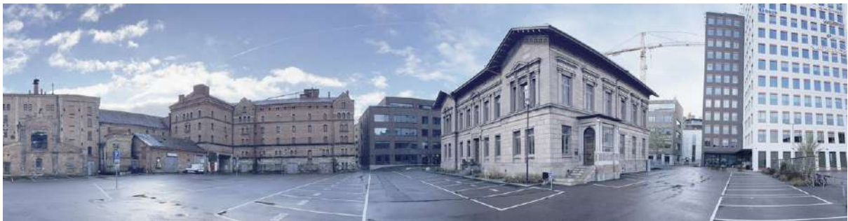
Image 21. Panorama view from the eastern side, highlighting the relationship between the manager's house and brewery structures.
