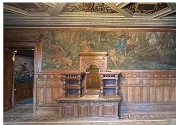
Image 59. The joinery, oak wall panels, and an original piece of furniture.
