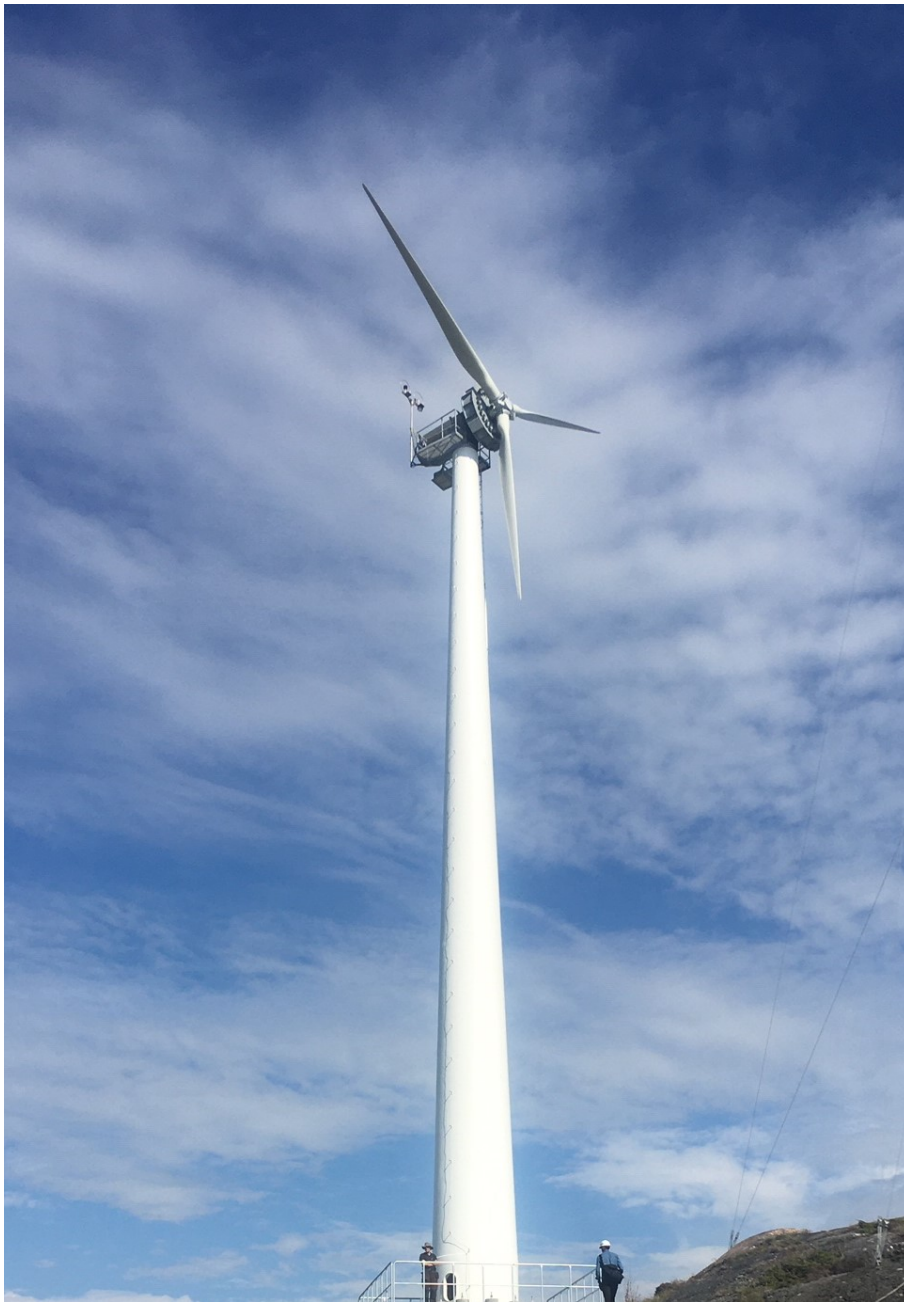
Figure 1.1: The Chalmers research turbine on Björkö with the prototype wooden tower made by Modvion.
