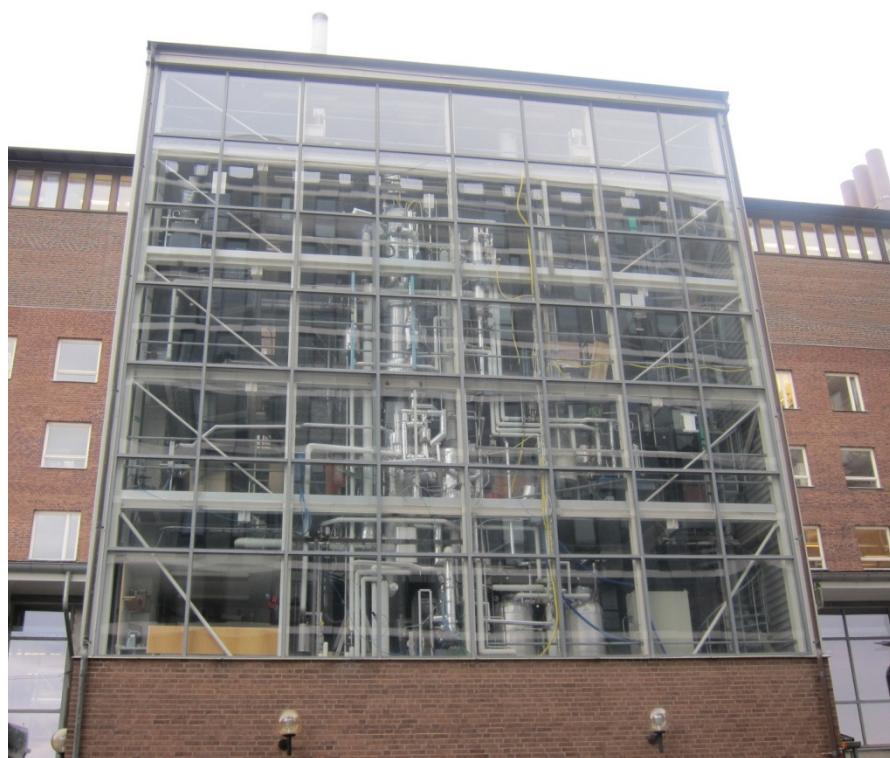
Figure 3.1 The evaporator pilot plant from outside the facility.
