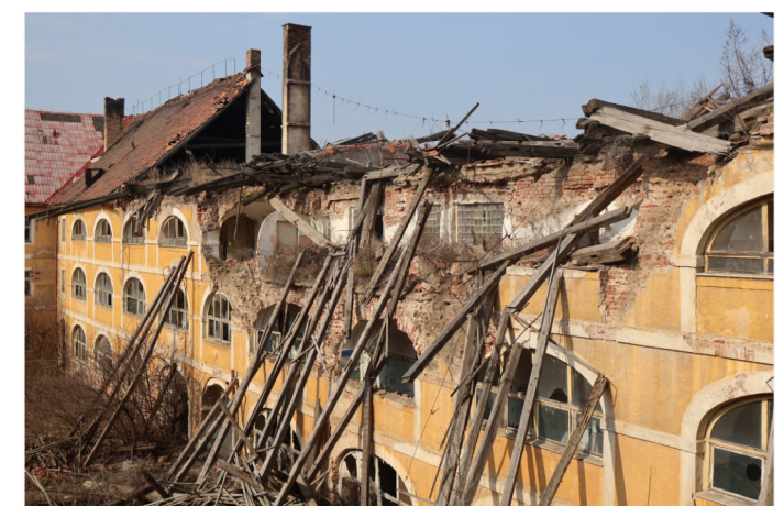
Figure 52: A collapsed section of second floor corridor wall and roof. The Dresden Barracks is in a constant state of deterioration
