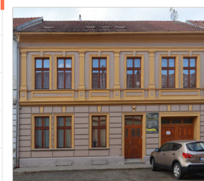
Electrician / apartment Mass dormitories
