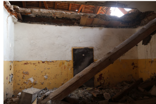
Figure 39: The ceilings of many spaces on the second have collapsed, revealing the roofspace above
