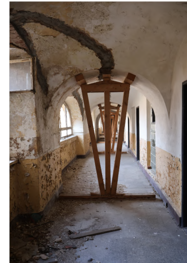
Figure 55: Structural supports in the barracks corridors
