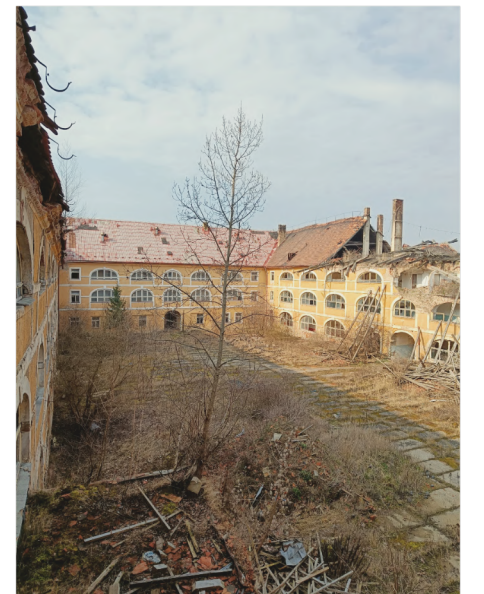
Figure 70: Central yard, current state
