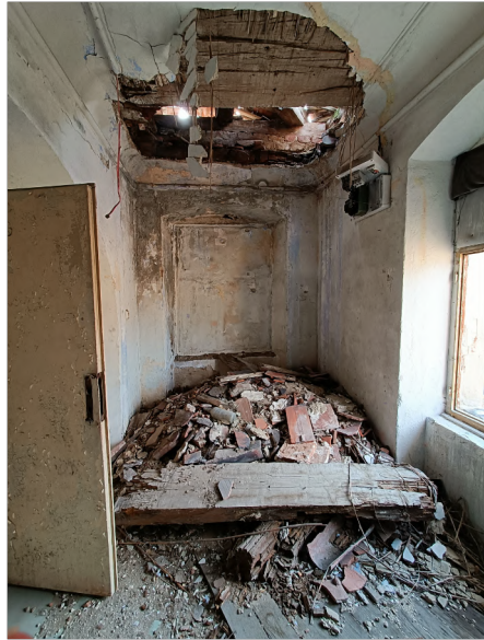
Figure 67: The former soldiers' chapel; both floor and ceiling will be removed to create a triple-height communal spiritual space
