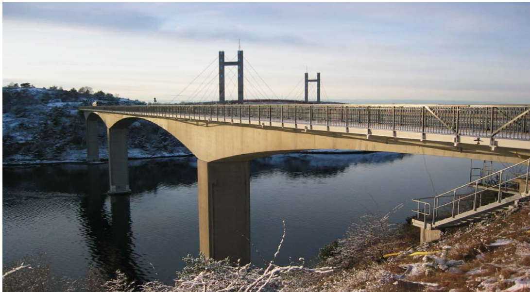
Figure 7.1 The Källösund Bridge seen from Stenungsöns, west direction. (Plos et al, 2004)
