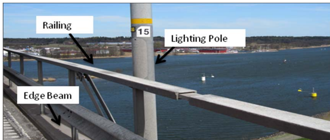
Figure 2.3. Edge beam supporting railing and lighting pole
