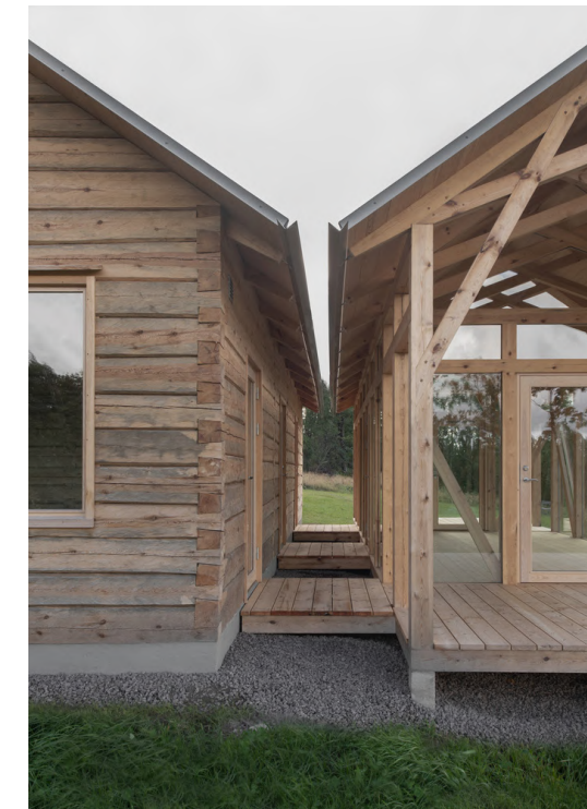
Figure 8 Timber frame and log structure. Photograph by Mikael Olsson, (n.d), from FABEL Arkitektur.
