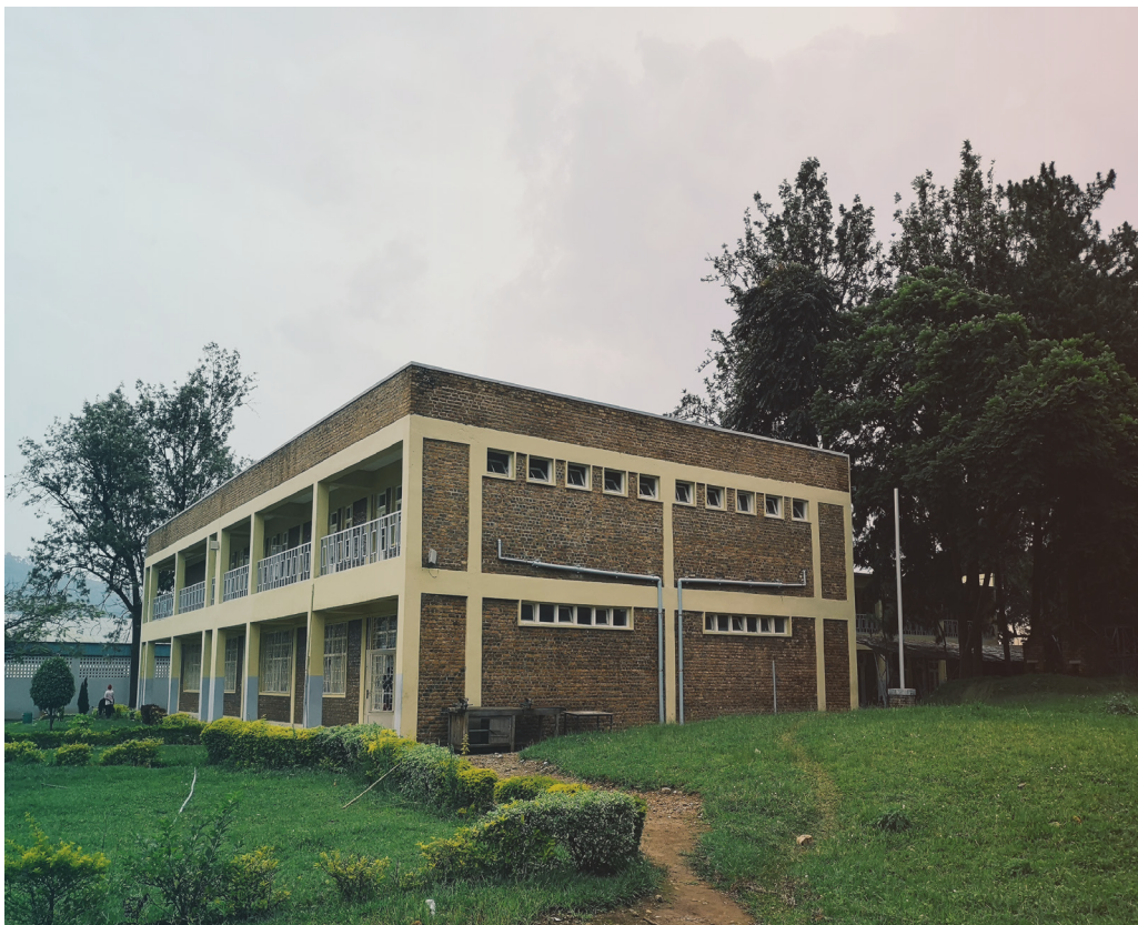
Figure 1.17. The back of the ACE-ESD Center building
