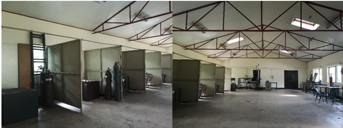
Welding Workshop, Nyarugenge campus, the University of Rwanda.
