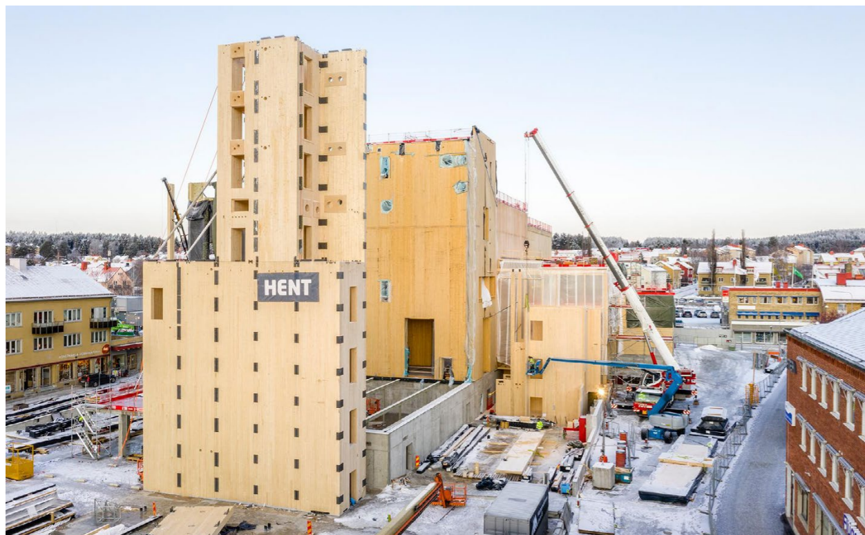
Figure 22. The wooden highrise Sara Kulturhus in Skellefteå during construction.
