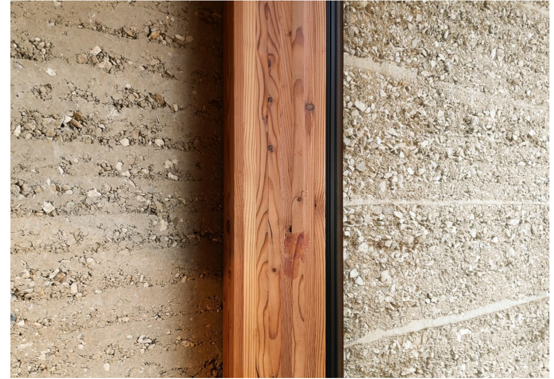
Figure 64. Interior and exterior. Swiss Ornithological Centre, Sempach.
