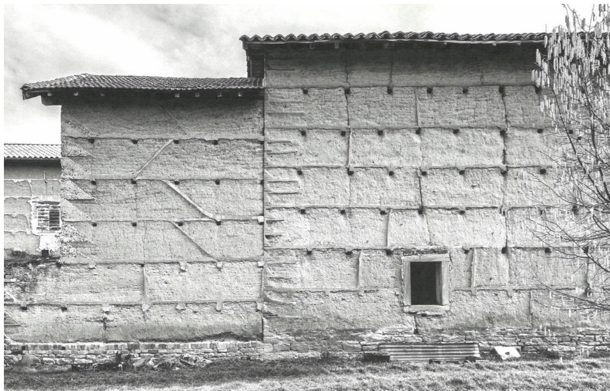
Figure 7. Old rammed earth barn in France, approx. 150 years old.
