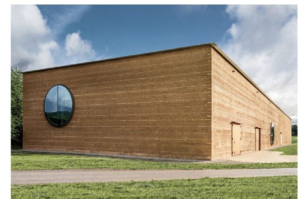
Figure 14. The finished result of the Ricola Herb Centre, made from prefabricated elements.
