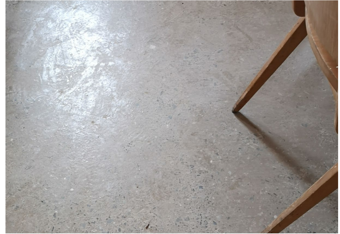
Figure 79. A polished and waxed rammed earth floor. Erden Werkhalle, Schlins.
