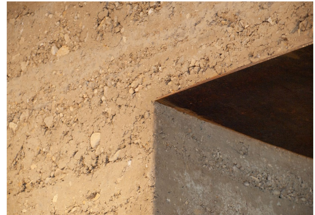
Figure 82. A thin metal plate seems to support the earth above, but a lintel beam is hidden behind. Swiss Ornithological Centre, Sempach.
