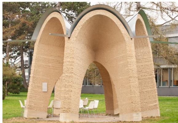
Figure 15. The ETH Cupola is a compression-only structure.
