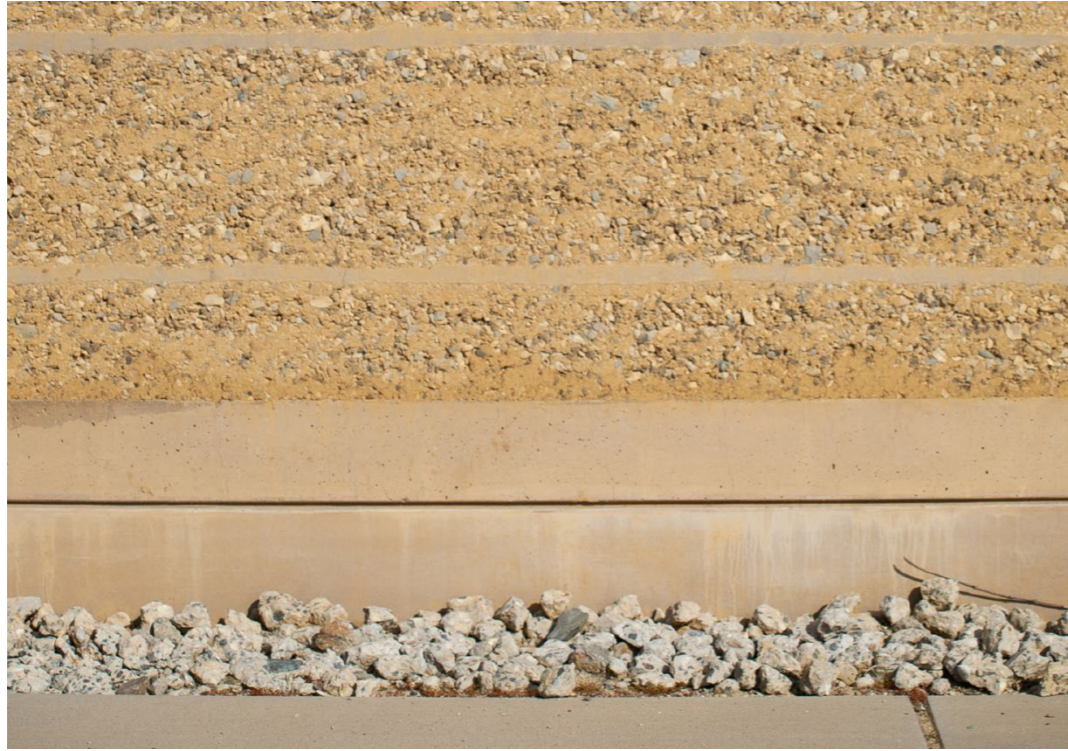
Figure 83. A patch of stones is placed below the facade to hide any eroded material coming from above. Alnatura Campus, Darmstadt.
