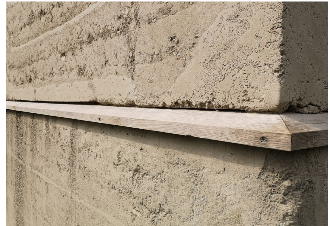
Figure 75. The wooden panels that these elements were prefabricated on were kept as erosion checks. Kiln Tower, Cham.
