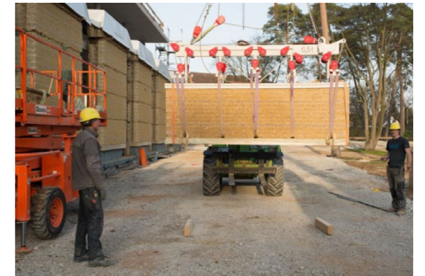
Figure 12. Lifting the elements on place with a crane.
