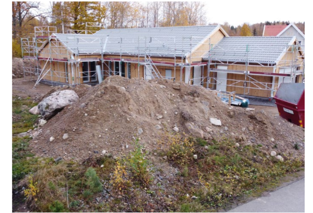
Figure 30. A pile of excavated earth next to a newly constructed house in Brokind.
