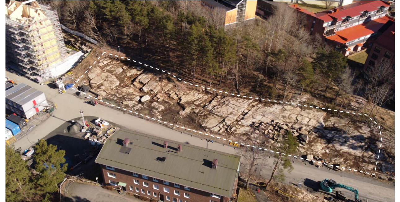
Figure 90. The site is located in a construction area and the topsoil over the bedrock has already been excavated.
