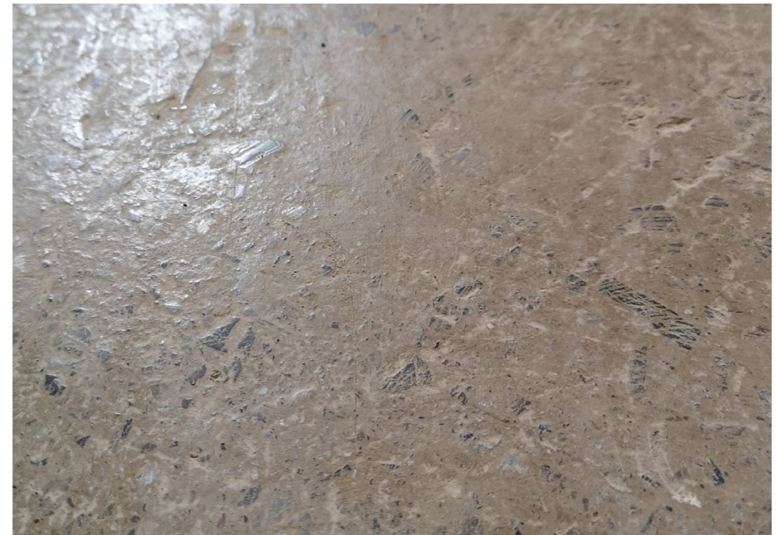
Figure 80. The appearance is similar to a polished concrete floor, but this has more roughness. Erden Werkhalle, Schlins.
