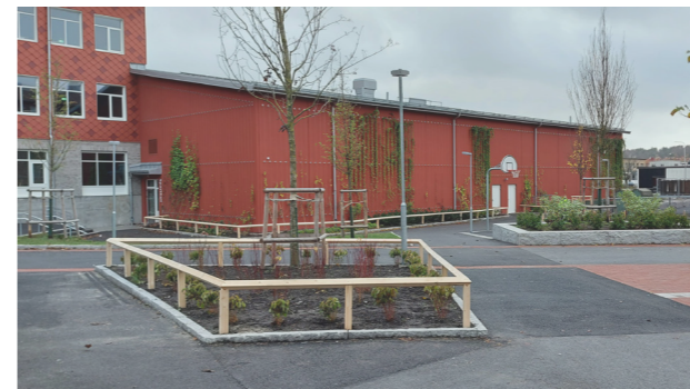
South school yard / Fenced greenery.
