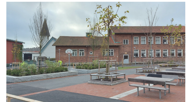
South school yard / Seating area, fenced greenery.
