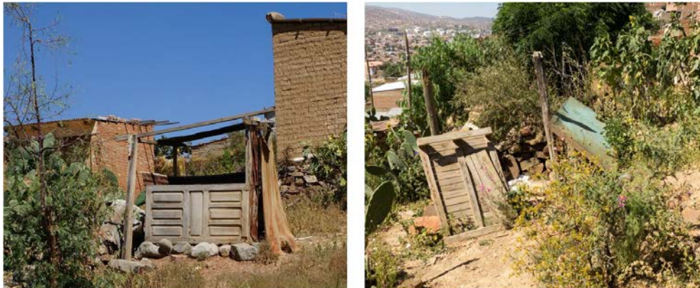
Figure 6.5 Two different unimproved pit latrines in the Study Area (Photos: private)
