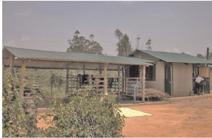
Figure 32: Gasifier shed with fuelwood storage and processing shed attached (Buchholz, et al , 2012).
