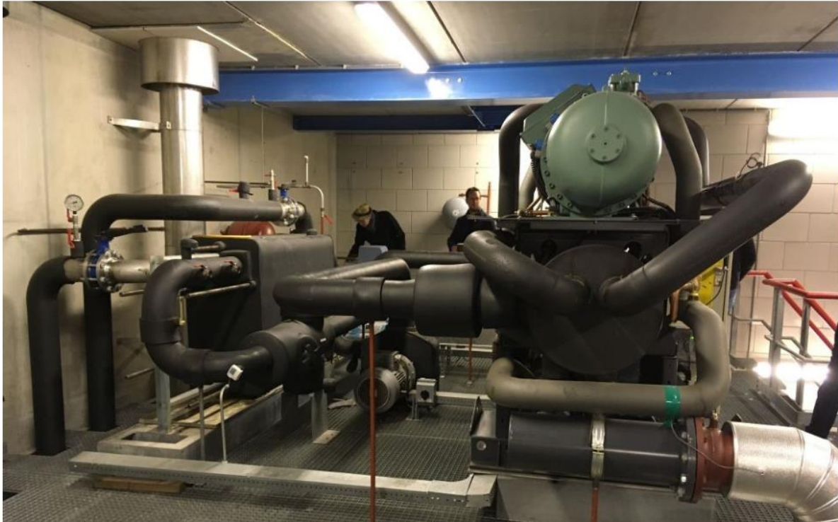
Figure 2.3. A photo of the oldest TED installation in the Netherlands, including a heat exchanger (HE) (left) and a heat pump (HP) (right), that is owned by an energy corporation and extracts heat from a drinking water company's clean water reservoir. (Figure from KWR, 2022).
