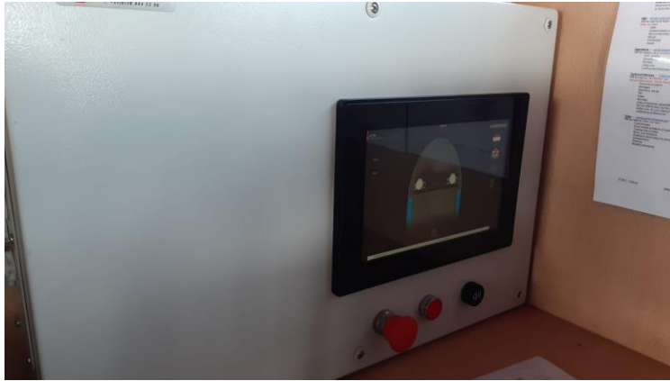
Figure 19. Software on bridge where crews put the units automatically up and down (Source: Van Dam Shipping)
